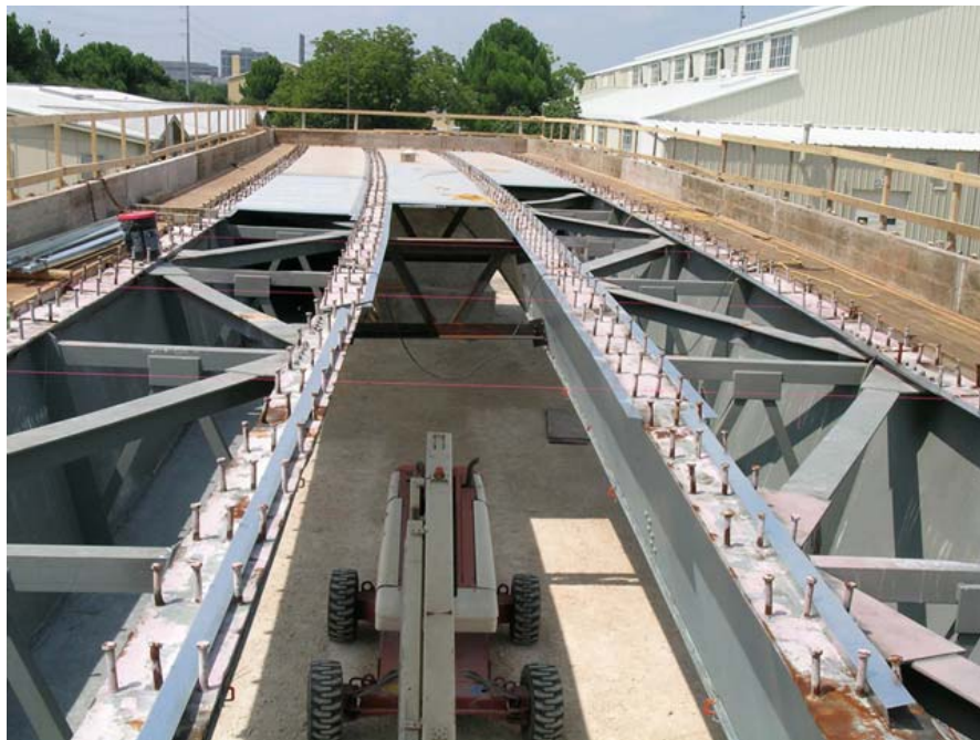
Figure 1-3 Internal Bracing System
